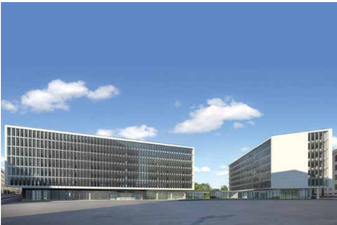
Figure 9 – Portuguese pilot building (left), EDP headquarters
